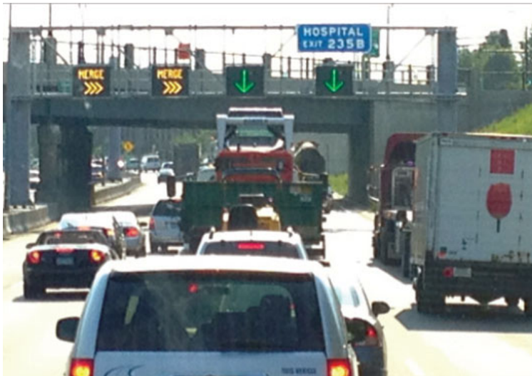
Using ATM for lane closures on I-94 in Minneapolis (Photo Courtesy FHWA)
