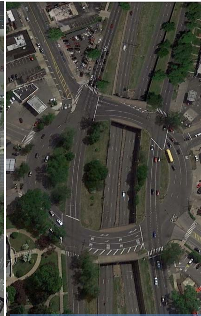
US 1/13 Philadelphia Signalized Traffic Circle
